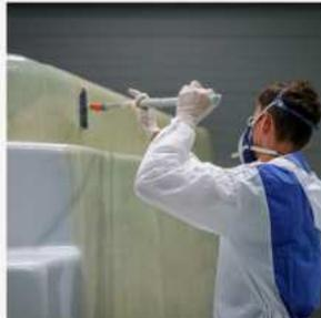
3. Application of an anti-corrosion fibreglass cloth
